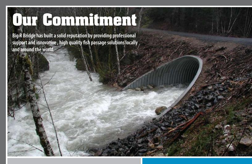
Big R Bridge offers a variety of fish passage structures to suit any application. Our open-bottom structural plate arches, box culverts and modular steel bridges can eliminate fish barriers by restoring the natural streambed. Structural plate boxes and arches are available in either galvanized steel or aluminum. Modular bridges can be fabricated as weathering or painted steel.
