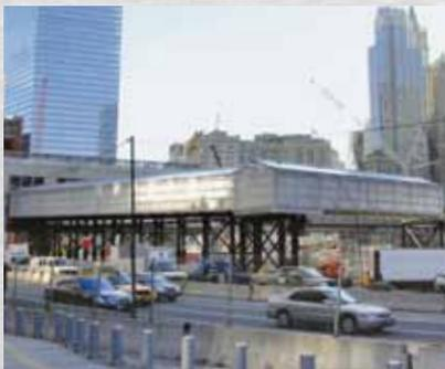
Our collaborative effort on this accelerated design-build project had to fit perfectly onto existing foundations. The contractor assembled and set the bridge in less than three hours, commenting that they had never seen such a perfect fit. Translucent paneling was requested to keep the busy route from becoming a viewing platform.
